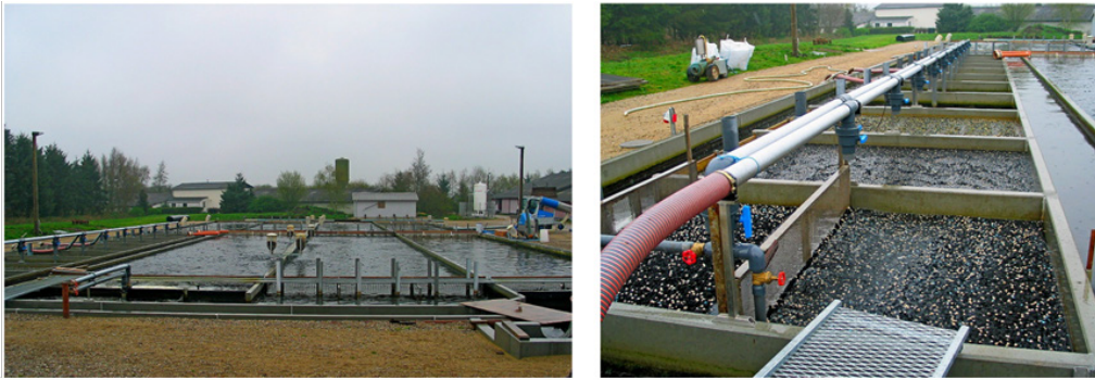
Figure 20: Grow-out phase of rainbow trout production in RAS: raceway concrete ponds, biological filters
